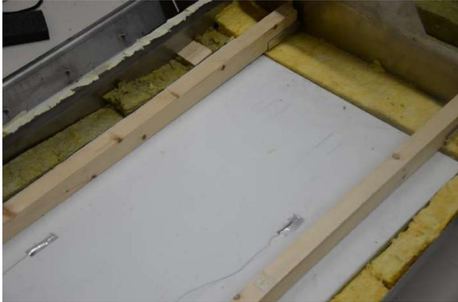
**Figure 4-12. Wooden support parts installation**
