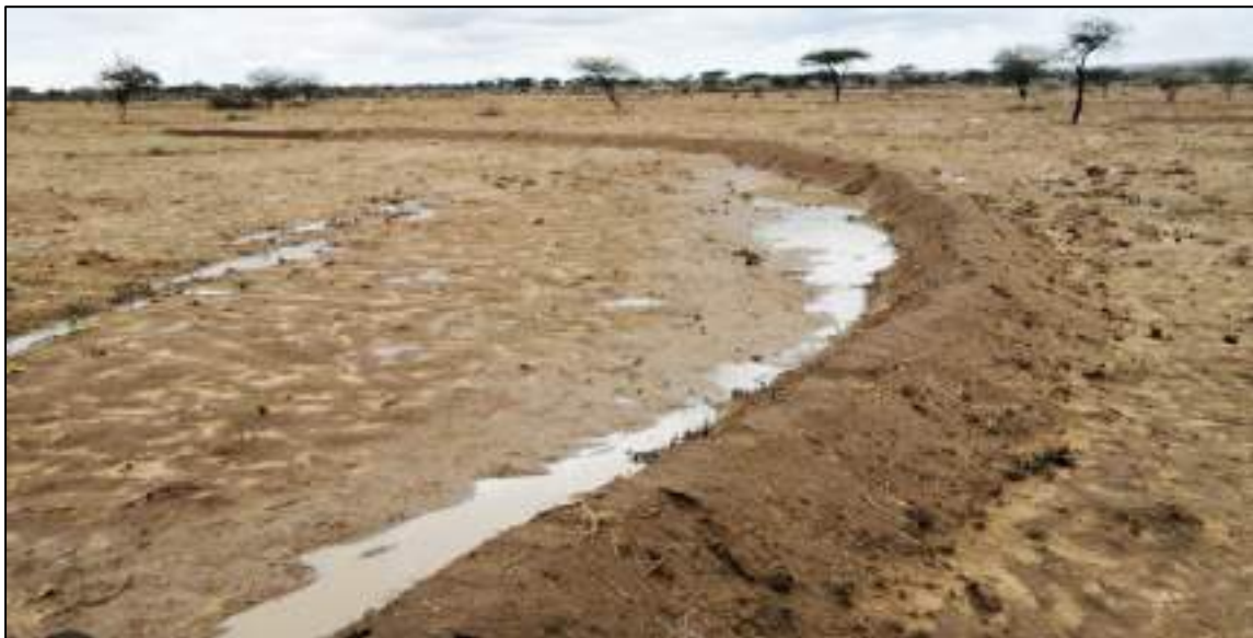
Figure 25 Semi-circular soil bund
